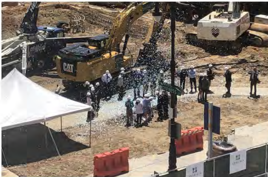
After general praise for the project at a Kimmel Center ceremony, the assembled dignitaries went across Broad Street to the construction site for the ceremonial groundbreaking. Those participating included developer Carl Dranoff; former Gov. Ed Rendell, who was mayor when the Avenue of the Arts project was launched; Mayor Jim Kenney; John DeFaroni, the original
